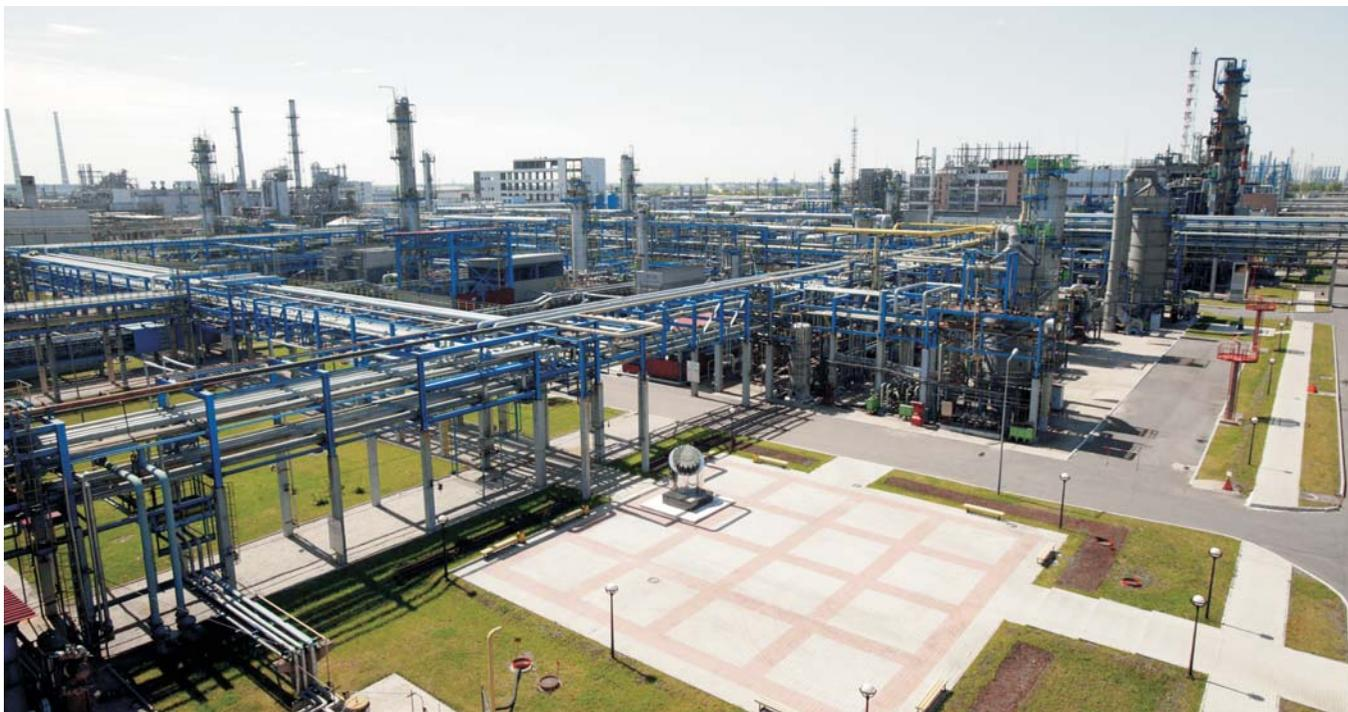
**TAIF-NK is constructing now three plants to produce high octane components for the motor gasoline plant: two of them – for MTBE production and etherification of catalytic cracking light naphtha by methanol, will be put into operation in the current year.**
